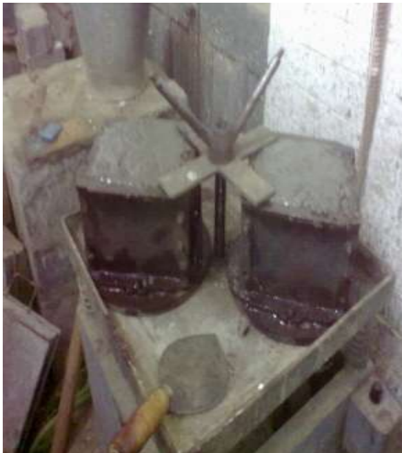
Fig.03 – Compaction of concrete (vibration)
